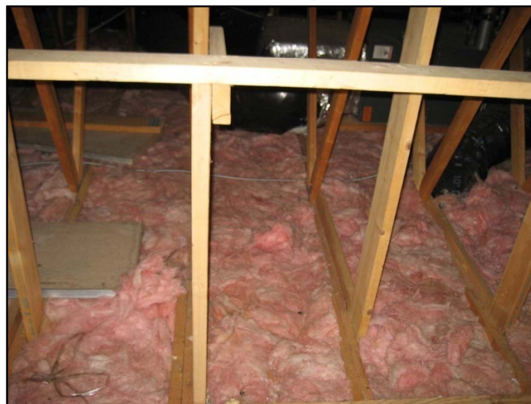
Photograph 7: Fiberglass insulation in convenience store attic.
