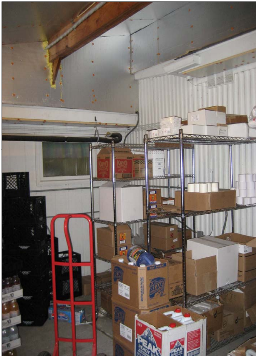
Photograph 5: Storage area showing fireproofing foam.
